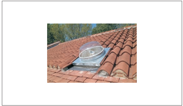
Figure 5 Curb mount installation
