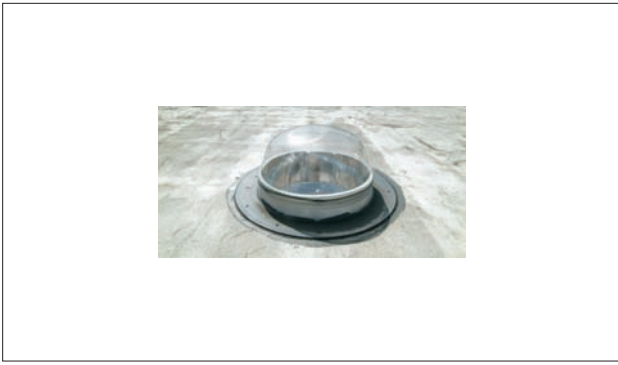
Figure 4 Flat roof flashing installation
